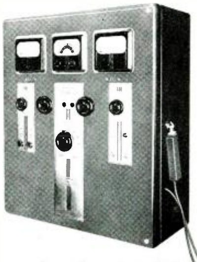
Control panel for an X-ray-fluoroscope unit.
